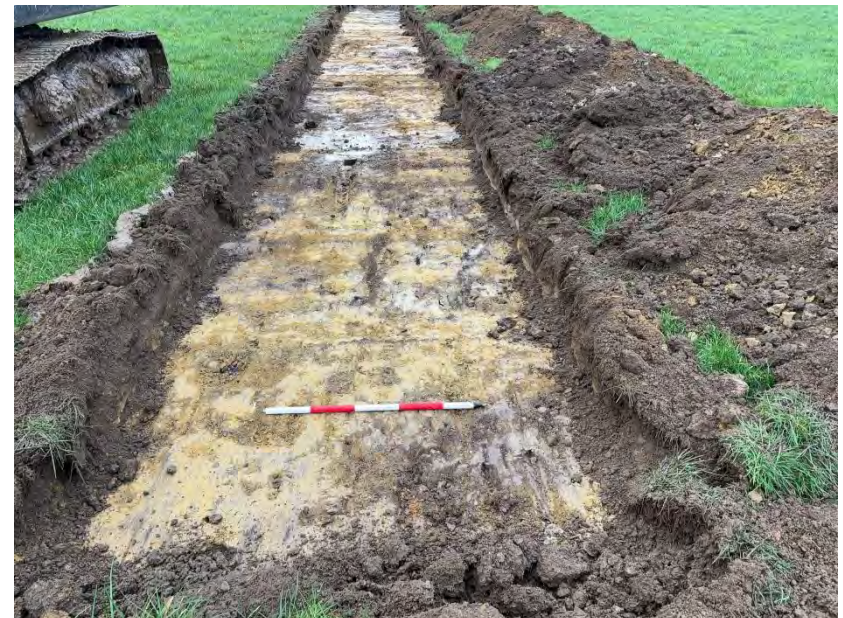
Plate 56: Trench 52 facing northwest
