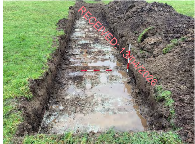
Plate 70: Trench 65 facing north
